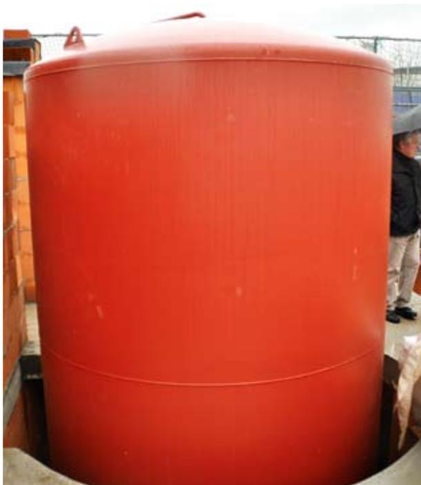
**Installation of a storage tank for a single family solar house inside the building envelope – this way, the heat loss of the tank is helping to keep the building warm.**
