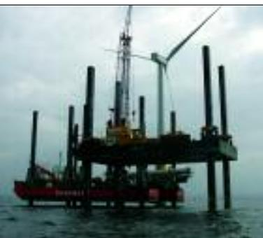
The »Annegret« barge and the Seacore jack-up installed nearly the whole North Hoyle offshore wind farm.
