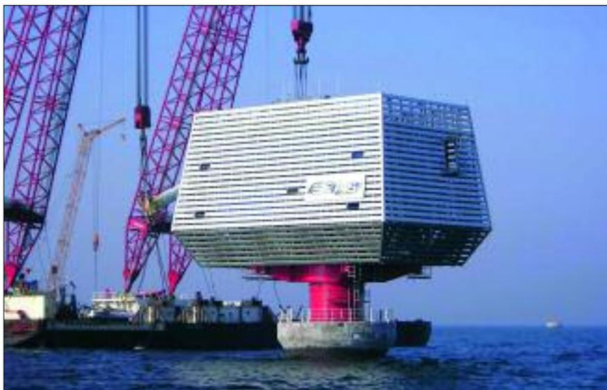
**Bladt Industries produced the platform for the 132 kV transformer station of the Nysted offshore wind farm.**
