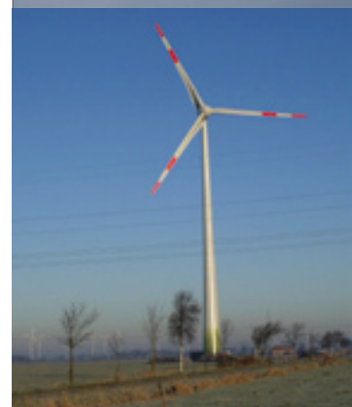
A further development from 2006: The Enercon E-82 has a rotor diameter of 82 m.
