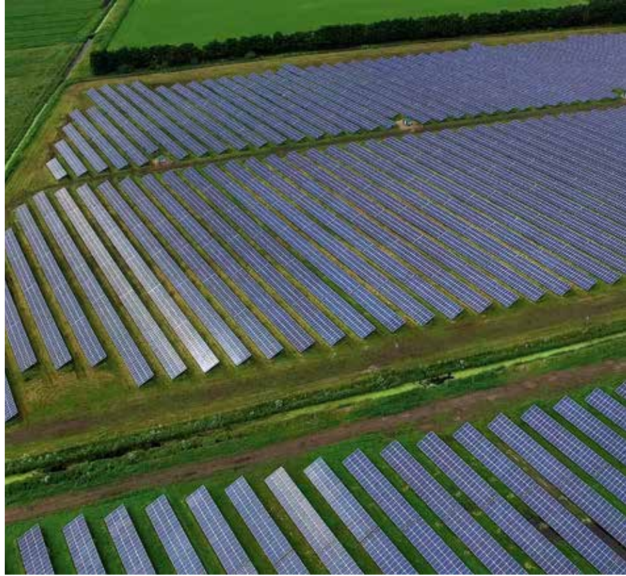
This 12.8 MW PV plant at Toggam Farm in the UK uses Huawei FusionSolar.
